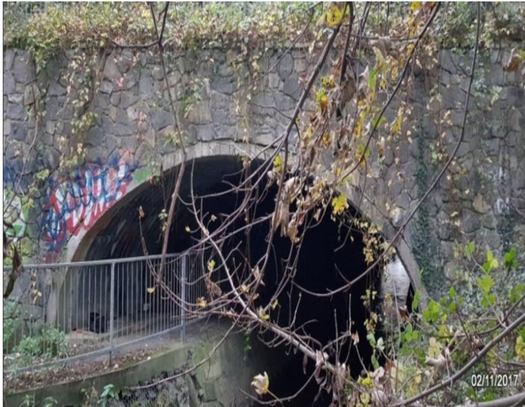
Figure 12: B31 Blanchardstown Bypass Bridge 1
